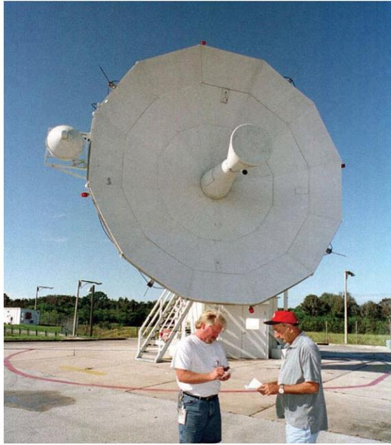
Above, the 9-meter antenna communicates with the shuttle orbiter during launch, in low-Earth orbit and during landing.
