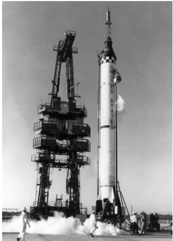
Preparations for the launch of Alan Shepard aboard a Redstone rocket from Complex 5 at Cape Canaveral.
